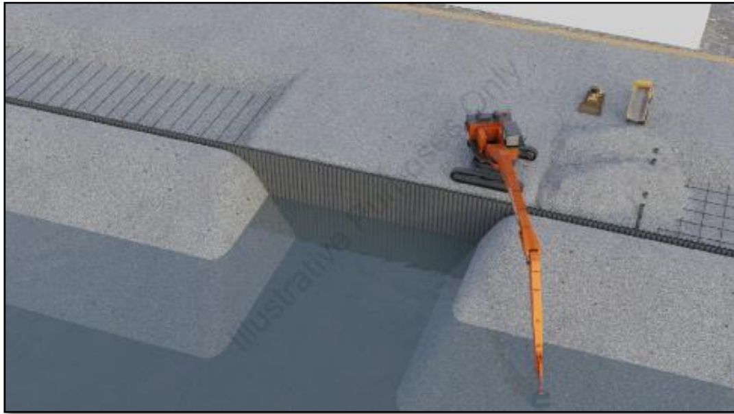
Plate 2-7: Schematic depicting removal of temporary working platform and backfill of tie rods
