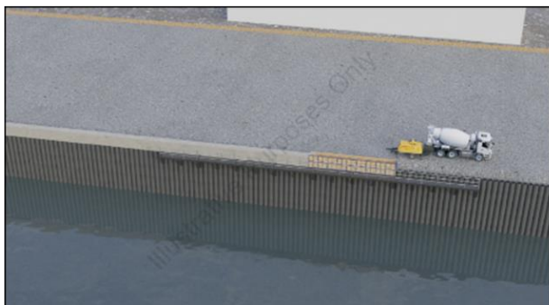
Plate 10: Coping beam installation
