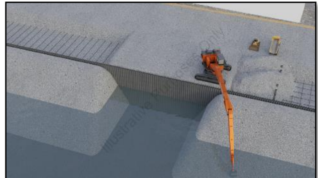
Plate 9: Removal of temporary working platform and backfill of tie rods
