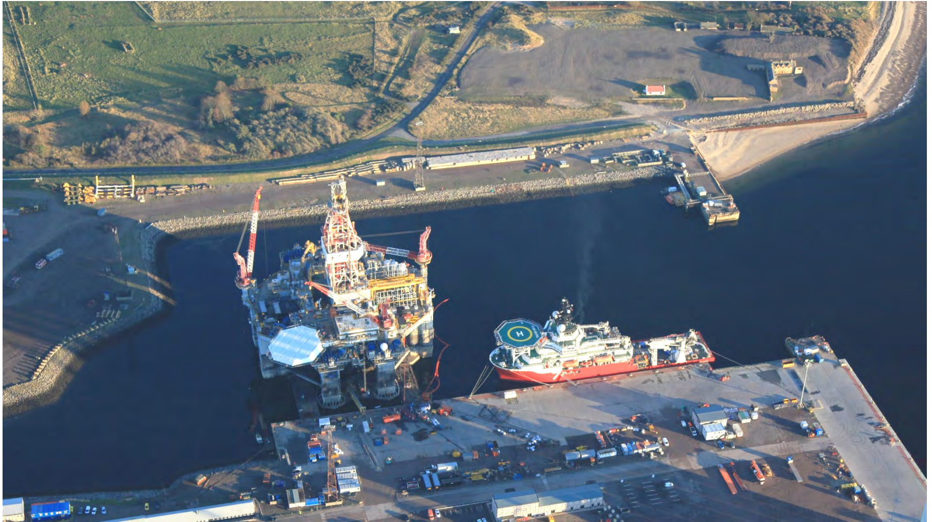
Aerial view from the West
