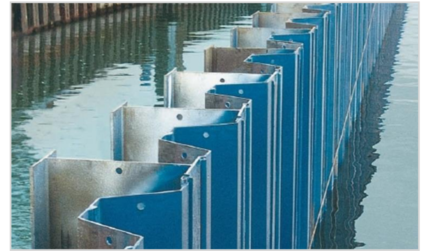
Example of sheet piled quay wall
